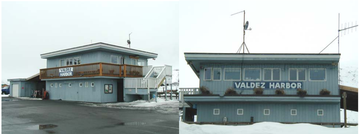
Valdez Small Boat Harbor Office with Attached Shop
