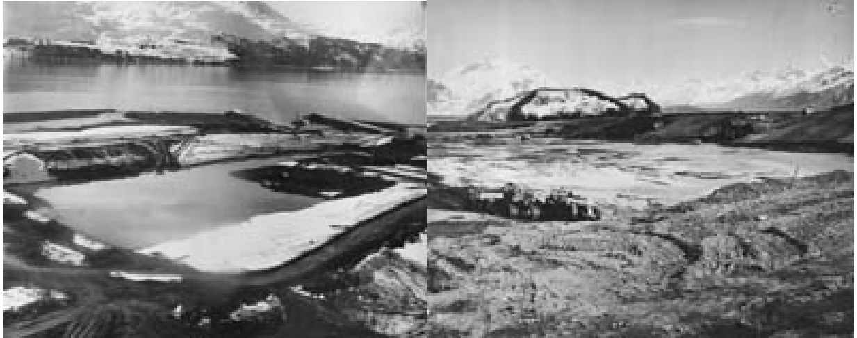
Construction of new harbor in 1965
